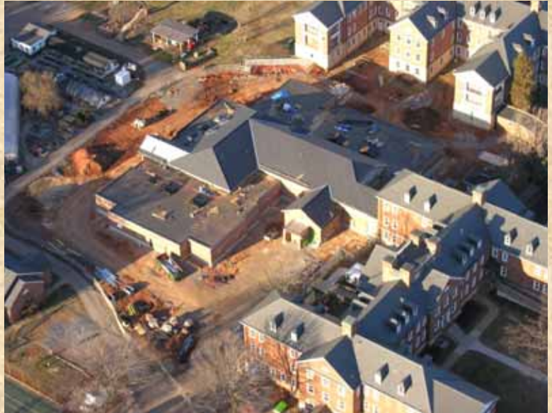
Aerial view of Building 8 Addition – Photo by Ricky May, SkyShots Helicopters.
